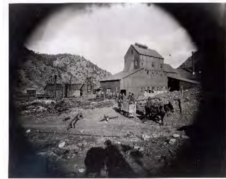
Stanley Mine photo courtesy of Christine Bradley
